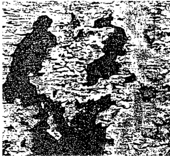
Fig 5.12 Severe Flaking
